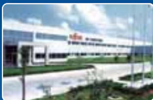
FUJITSU GENERAL (SHANGHAI) CO., LTD.
